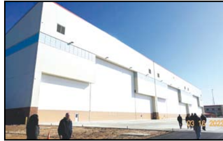
Travis AFB’s new aircraft maintenance hangar. US Navy photo by Tom Ishizue
