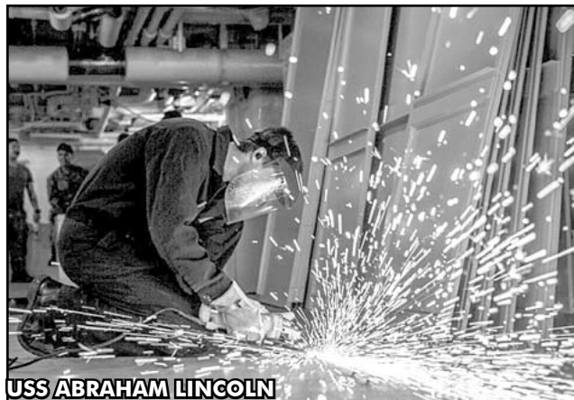
Navy Petty Officer 3rd Class Eagan Tate grinds down a stud as part of a rehabilitation project June 27, 2023. U.S. Navy photo by MC3 Thaddeus Berry
