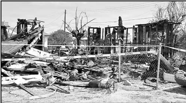
TWENTYNINE PALMS (Aug. 24, 2026) A home here shows extensive damage, following an explosion and fire. Navy hospital corpsmen and Marines responded to the incident, helping rescue two injured residents, evacuate neighboring homes and provide medical assistance until civilian emergency responders arrived. U.S. Navy photo by Christopher Jones
